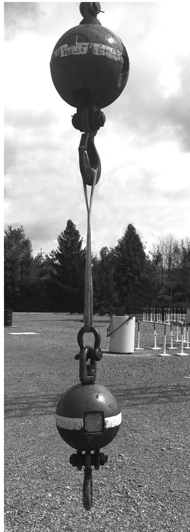
Rigging for Second Overhaul Ball (Task 3 Only)
