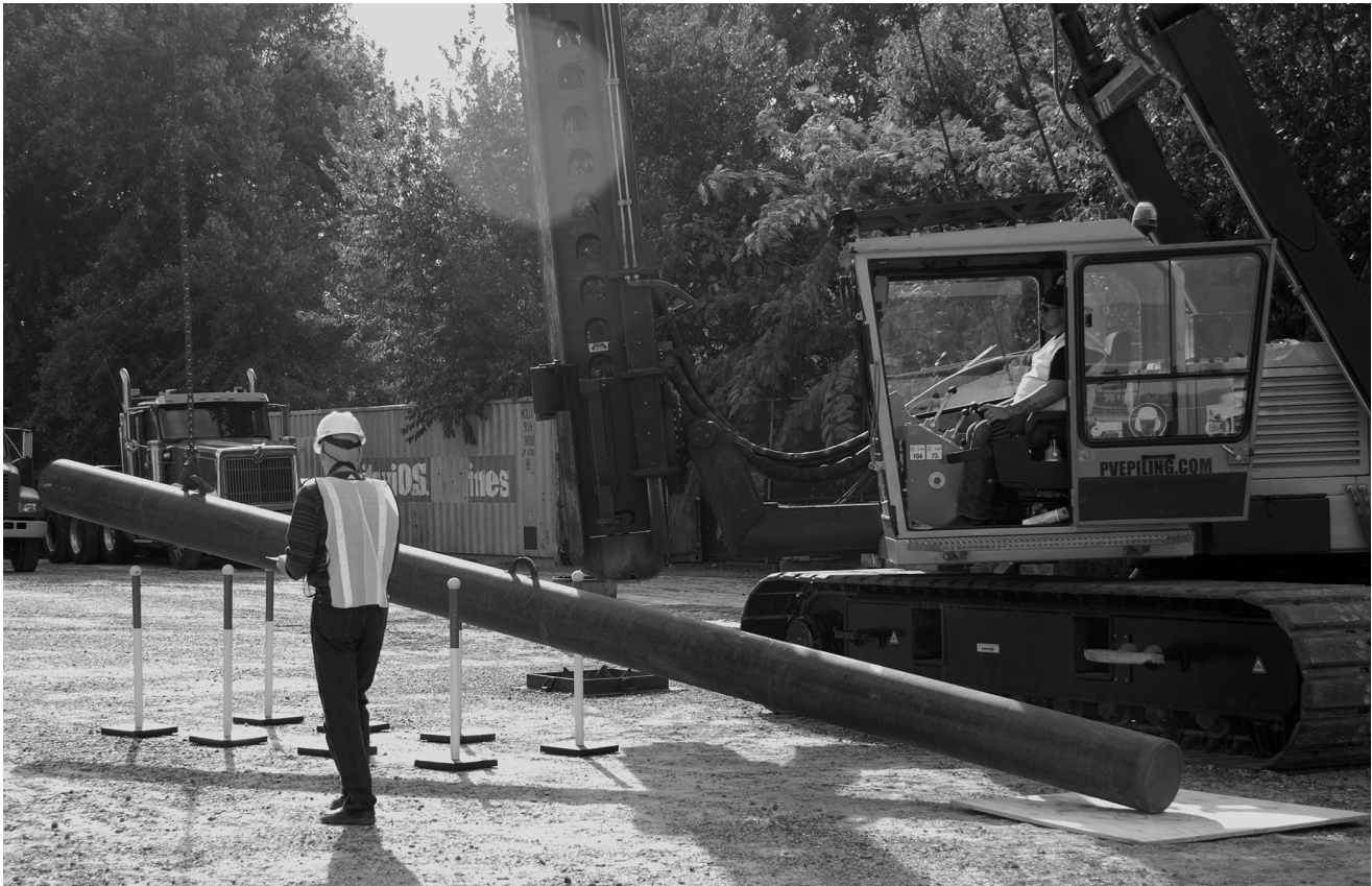
Test Pile (with 2 attachment points)
